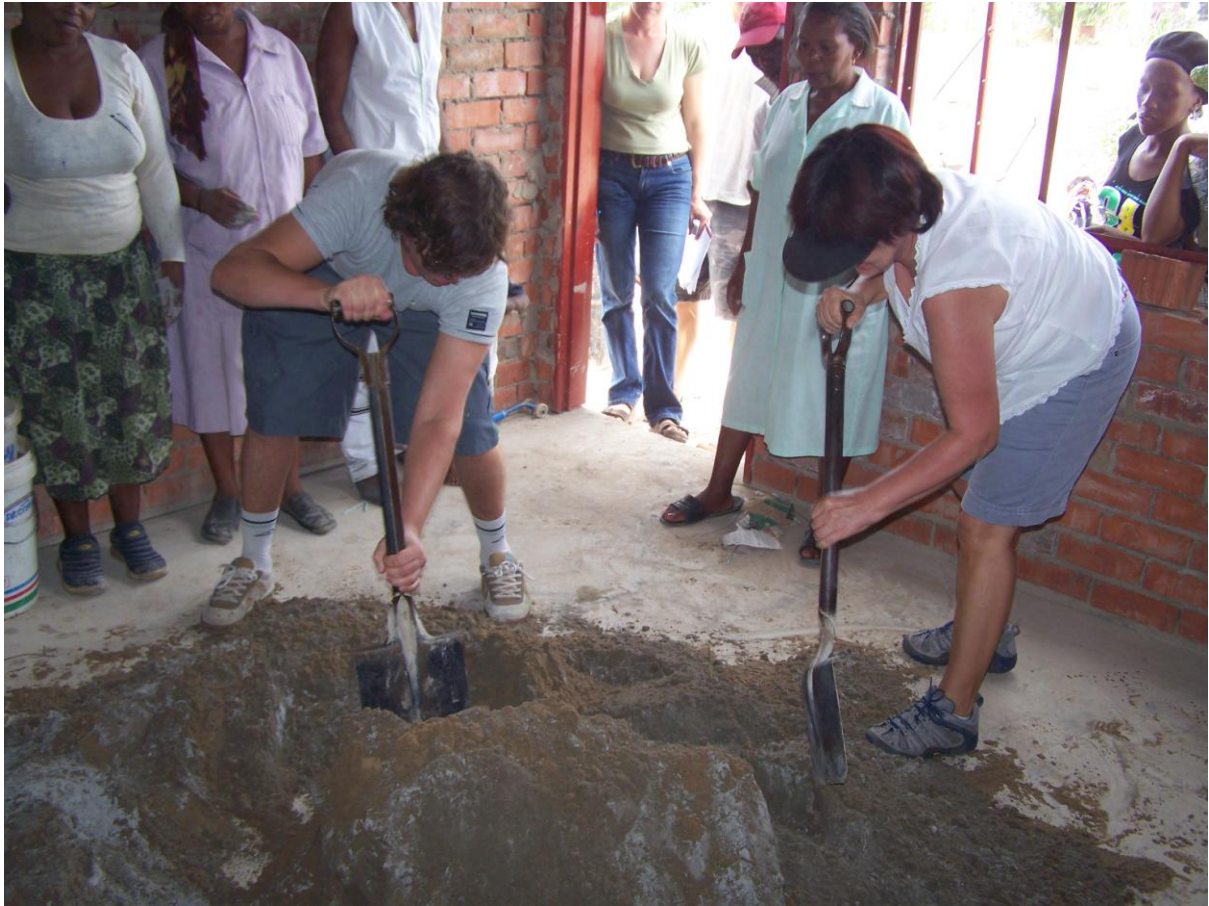
Time to start plastering the walls with a little help from students and the lecturer!!
